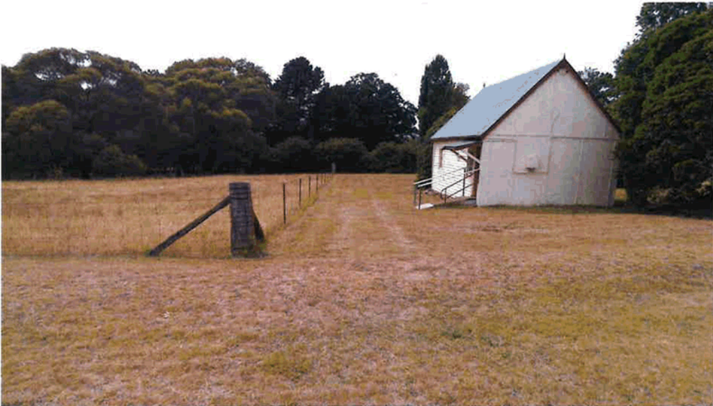
Photo 13 The fence line which is nominally 7m behind the Church. The proposed court extends some 17m beyond the fence line to the left above.
