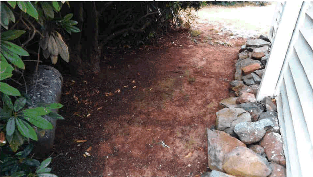
Photo 3 The gas bottle has been detached from the Church and left in the bushes. This hazard should be removed asap.
